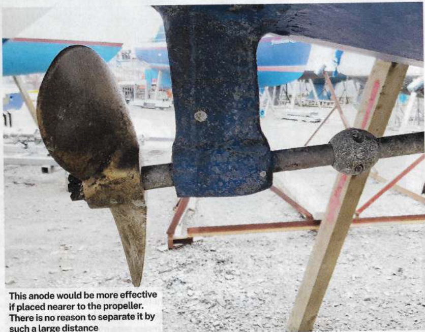
A propeller anode, secured with nylon screws to avoid excessive loss around metal ones, and a shaft anode attached close to the propeller. Anode life has doubled by painting the propeller, reducing the size of the cathode
