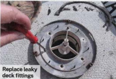
Check deck fittings for wear and tear
