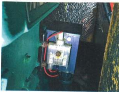
A fuse had blown but it wasn't affecting the alternator
