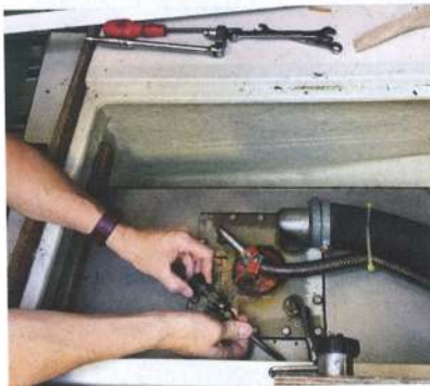
Undoing fuel lines ready to remove the inspection hatch of the fuel tank
