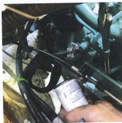
The secondary filter is removed
