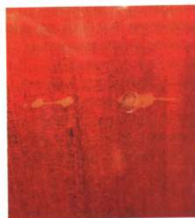
A scratch in the door turned ugly when moisture found its way under the lacquer
