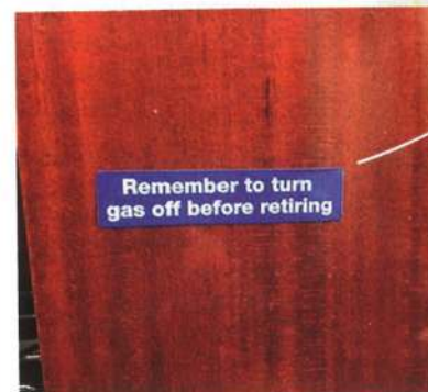
A scratch in the door turned ugly when moisture found its way under the lacquer
