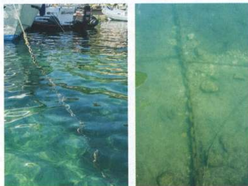
The bow line from each boat is connected to a chain. This in turn is connected to a bigger chain that runs parallel to the dock. The big chain is secured at either end to the dock or a large lump of concrete
