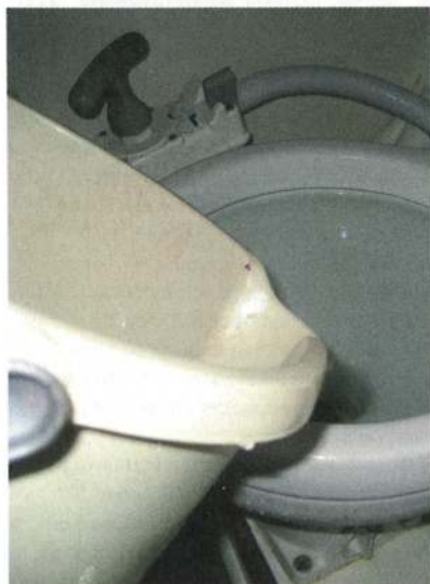
Start by flushing two buckets of fresh water through the system
