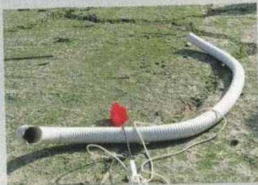
Drop a line through the pipe and use it to draw a bottle brush back and forth
