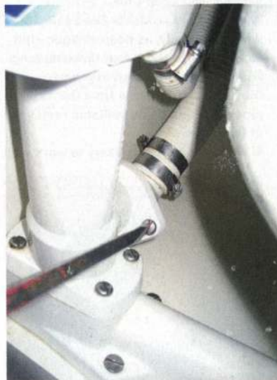
With foul water replaced with clean, joker valve is relaxed to empty the waste pipe
