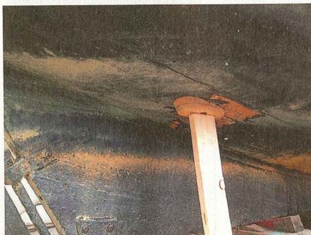
A tapered pad was bolted through the hull to level the motor fore-and-aft
