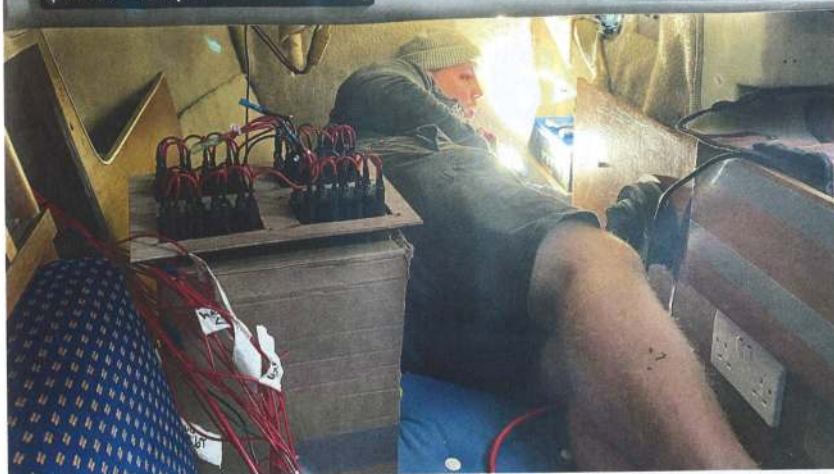
Installing the batteries aft under Maximus's cockpit
