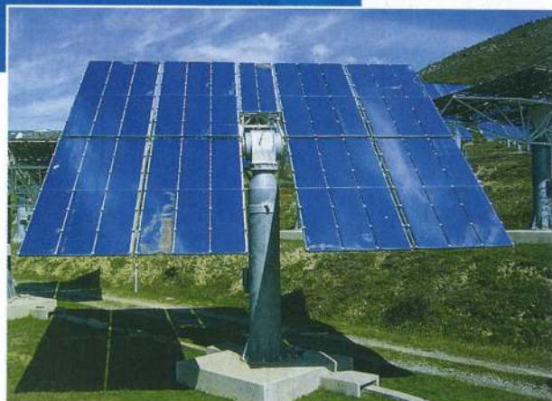
BELOW Two-axis tracking mounts allow solar panels to make the most of the available sun
