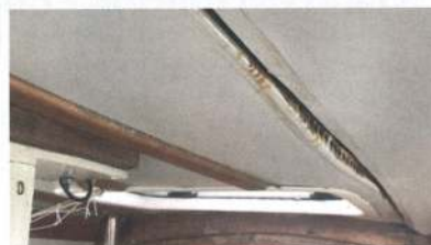
Surveyors won't dismantle headlinings, but removing this wooden batten revealed damage from water ingress that wasn't otherwise apparent
