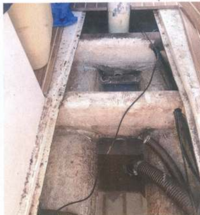
A dirty bilge, with inches of murky water, won't allow a surveyor to inspect the tops of the keelbolts properly
