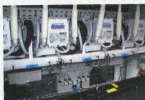
A bank of chillers serving a large motoryacht. Each chiller is assigned to an area of the yacht, much as in a hotel ashore. The temperature can be set locally on a bulkhead thermostat
